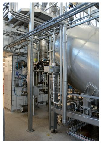
Sesotec metal detector P-SCAN RG installed in a vertical conveyance pipeline
