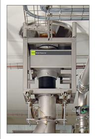
The RAPID 5000 operates as an effective metal detector for the inspection of powdery and fi ne-grained bulk materials. It detects and rejects magnetic and nonmagnetic metal contaminants, with a unique elliptical stainless steel reject flap diverter. The leading hygienic design does not have any corners or niches that can be harborage areas for pathogen growth, making it suitable in applications where high sanitary standards are required.
