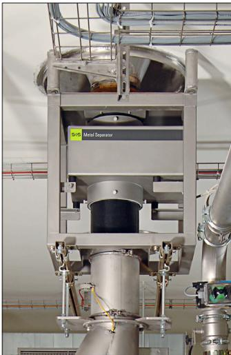
The RAPID 5000 operates as an effective metal detector for the inspection of powdery and fine-grained bulk materials. It detects and rejects magnetic and nonmagnetic metal contaminants, with a unique elliptical stainless steel reject flap diverter. The leading hygienic design does not have any corners or niches that can be harborage areas for pathogen growth, making it suitable in applications where high sanitary standards are required.
